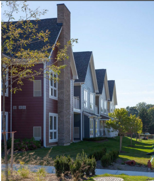
Figure 9 - This 28-unit apartment building in London, Ontario (77 Tecumseh Avenue) is designed to fit within a neighbourhood of single-detached homes and provides a housing type suitable for an aging population.
