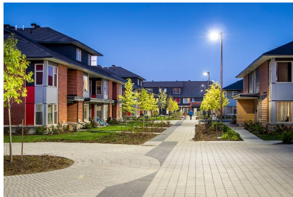
Figure 11- The Haven - Multi-Faith Initiative Housing in Barrhaven, Ontario. Hobin Architecture
